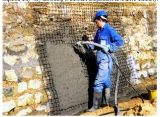
When spraying to a thickness over 100mm, care should be taken to ensure that the build up is not too rapid resulting in possible slumping, as large an area as possible should be worked. Avoid feathering edges by cutting back at least 10maround the area to be sprayed if required. Substrate movement joints should be continued through the Sprayfast layer and suitably sealed.
